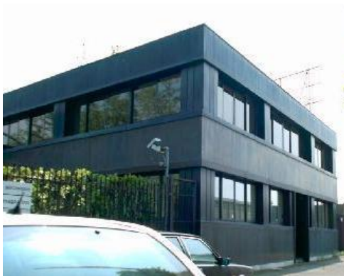
OxyTech Headquarters – Cornaredo (Milan, Italy)
